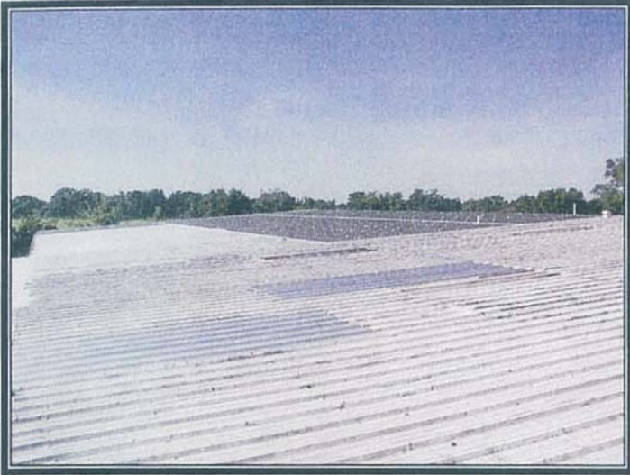
Building 7 – Roof – Typical of Majority of Roofs on Property – Prefabricated Sheet Metal
